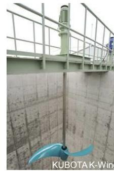
Fig. Mixer ad asse verticale – Kubota K-Wing
