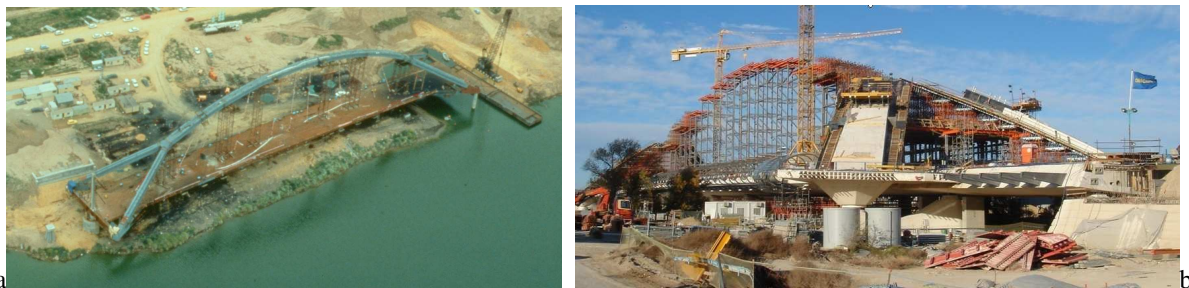
Figure 3. Construction methods. a) Barqueta bridge built on a river side. b) Third Millennium Bridge built on site with the continuous falsework
