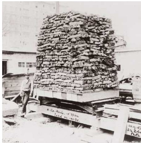
Figure 3: Load test on a vault performed by Guastavino, New York City, 1901.
