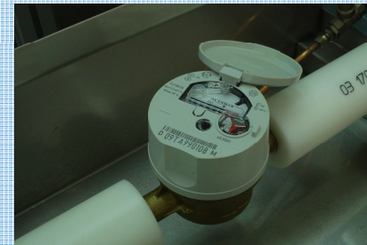
Class C; Q_3 = 1.5 \text{ m}^3/\text{h} ; DN 13 mm
