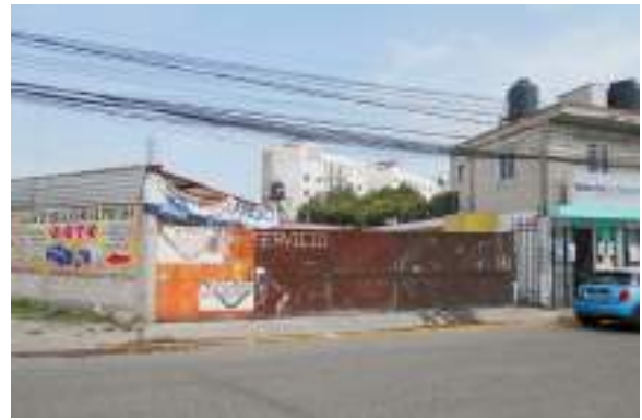
Fig. 6. Cholula, calle De la Mesa and, in the background, the recently built Vitale Residential (authors' photo).
