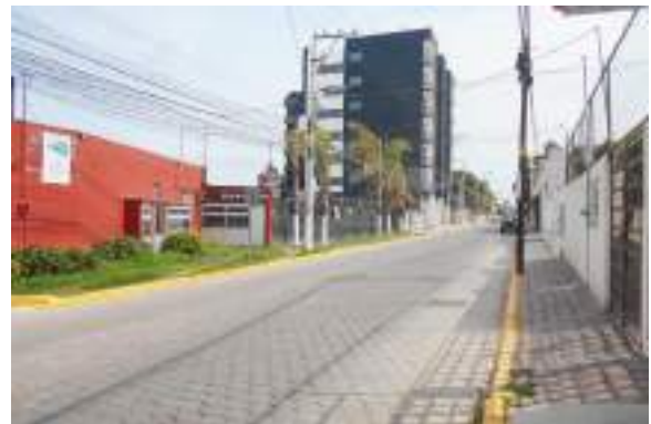
Fig. 7. Cholula, the ongoing seven-stories building in calle De La Mesa (authors' photo).
