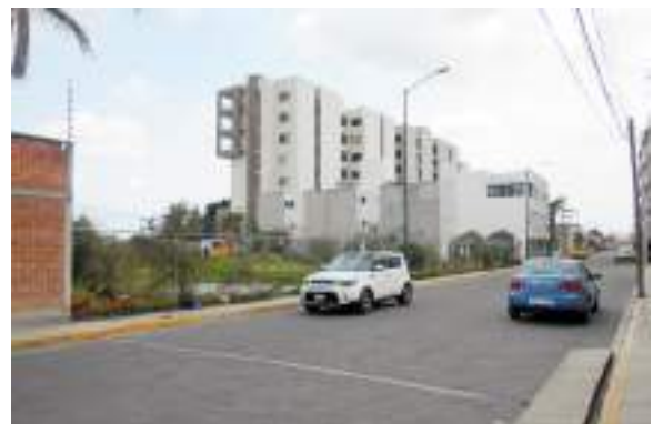
Fig. 8. Cholula, the ongoing eight-stories building in calle 10 Oriente (authors' photo).
