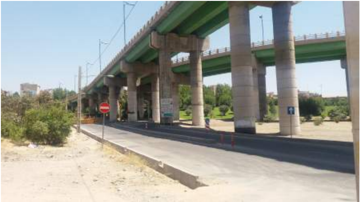
Fig. 3. Tehran, Niayesh Highway.
