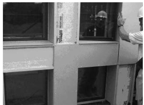
Installation of L-shaped aluminum panels.
